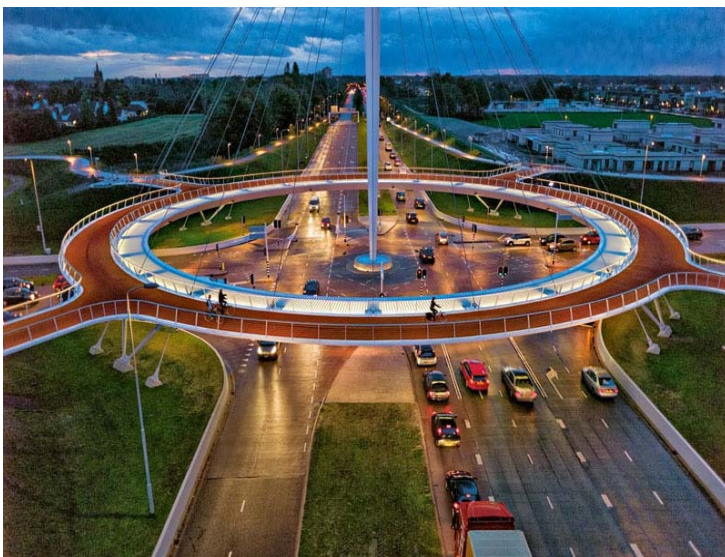
Photo shows the Hovenring, Eindhoven.
